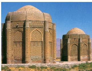
D: Kharaghan, Zanjan
