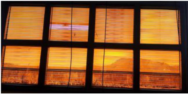
Fig. 8. DSSC PV wall system, made by Daunia solar cell.
