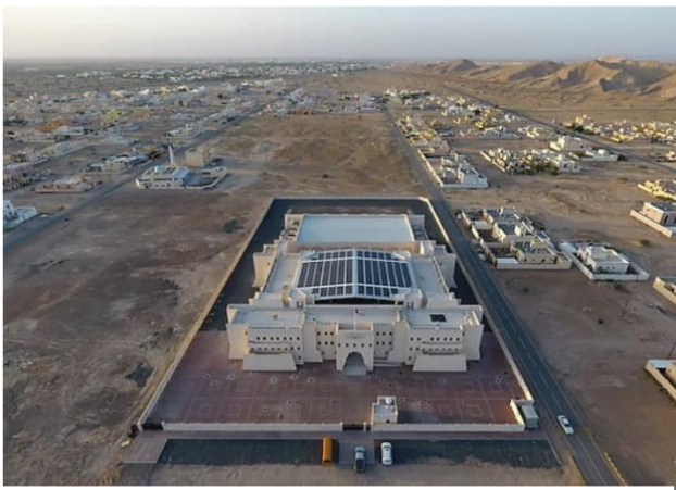
(b) Solar PV penetration in Kaab bin Barsha School
